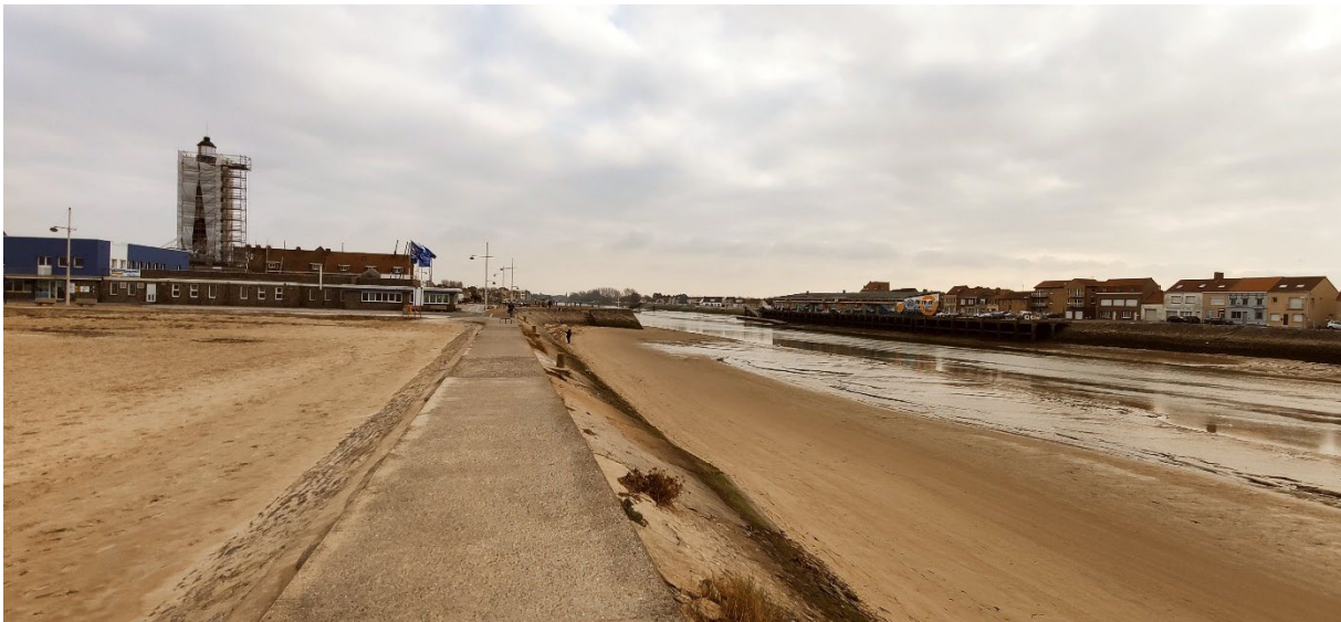
Figure 8: The lighthouse (under repair at the time photograph was taken) in relation to the canal and foreshore.
